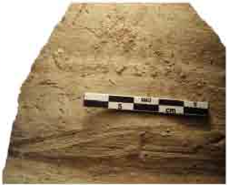
Logardan Technique 4: construction by overlapping flattened slabs of around 5 cm thick
