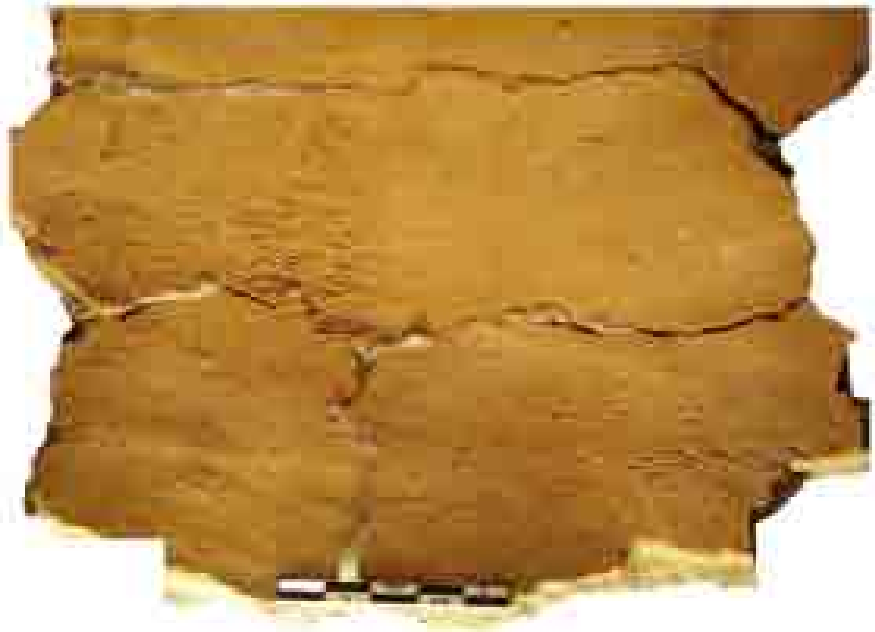
Logardan Technique 4: construction by overlapping flattened slabs of around 5 cm thick
