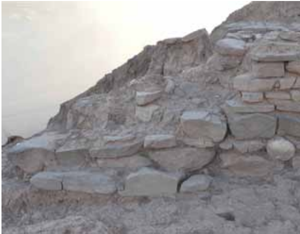
Fig. 7 - Level 4a - restructured portion of Wall 636.
